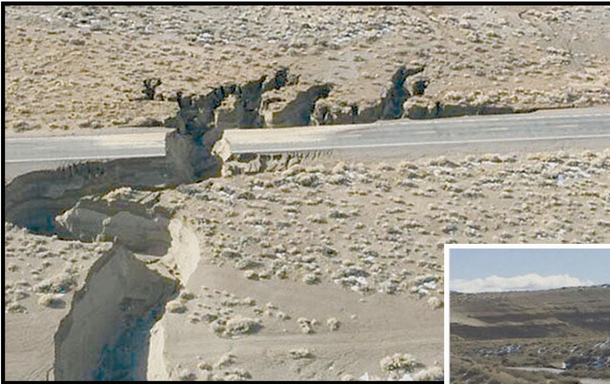
The runoff tore out a huge portion of SR446 that closed the highway for over a month.
