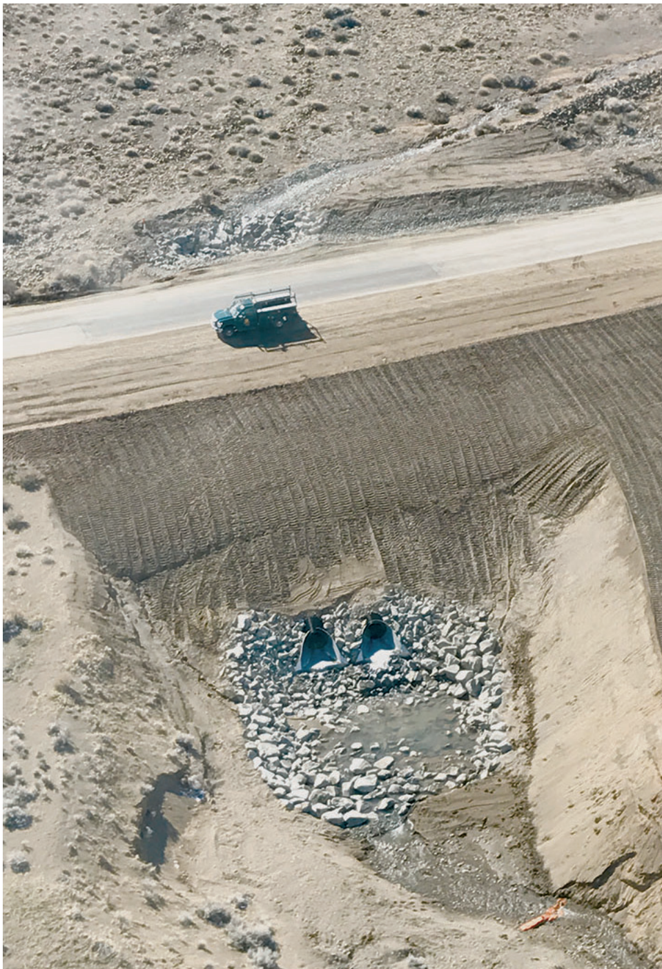
One of the sections of SR446 repaired by Granite Construction
