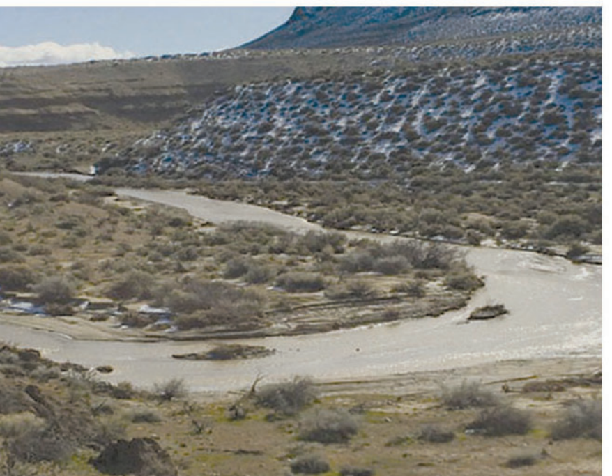
Mullins Creek caused major damage to the water supply serving Sutcliffe.
