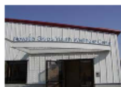
Finished Facility July 10, 2008
