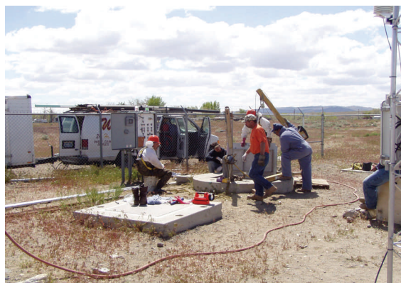
(Conducting repair work and unclogging the Wadsworth sewer lift station.)
